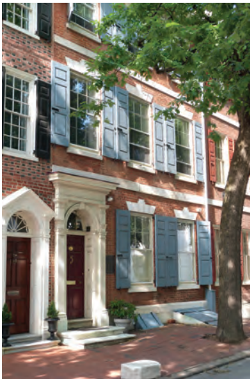
Williams-Mathurin House 427 Spruce Street
